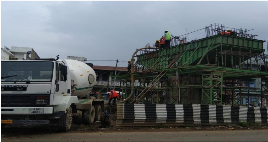
Pier cap Concrete P5 of LC-32
