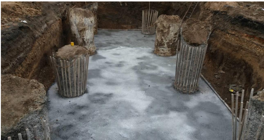
Pile cap PCC at LC-41 of Pier P2
