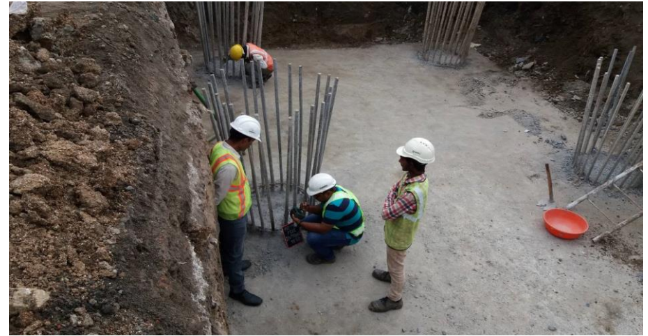
Pile Integrity Test at LC-41 for Pier P2
